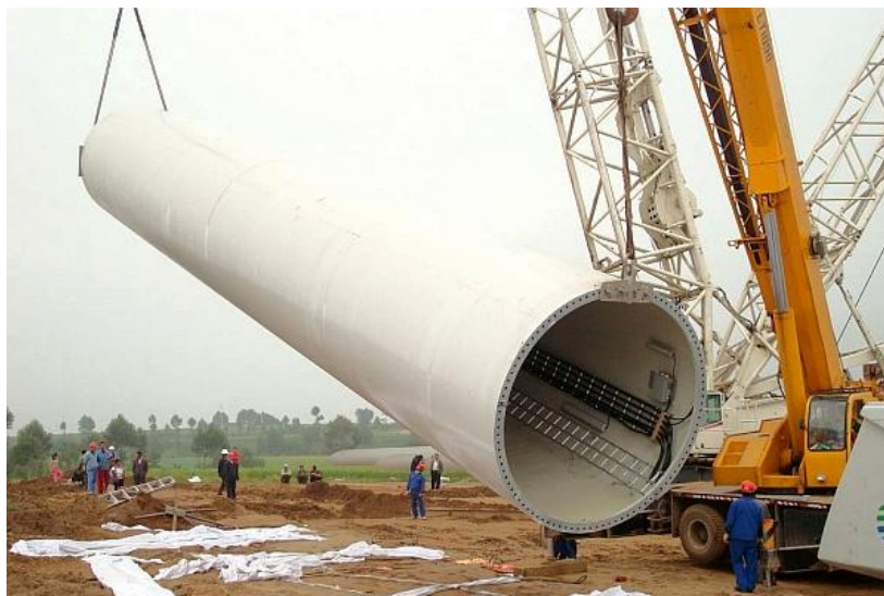
Installation of tower segments at designated site
