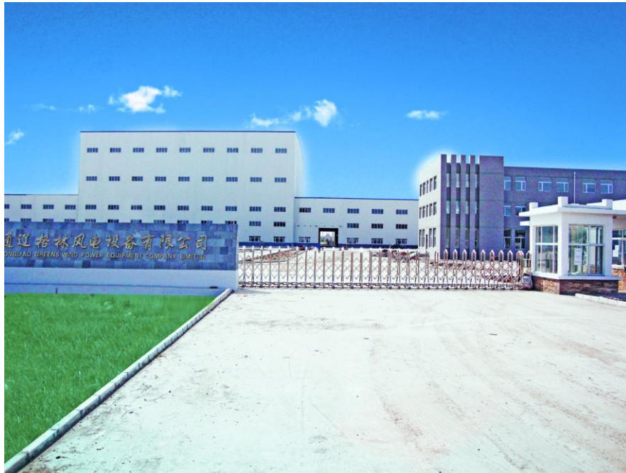
The newly completed plant in Tongliao City, Inner Mongolia, is an advanced facility for manufacturing steel towers located inside the biggest wind-farm in China.
